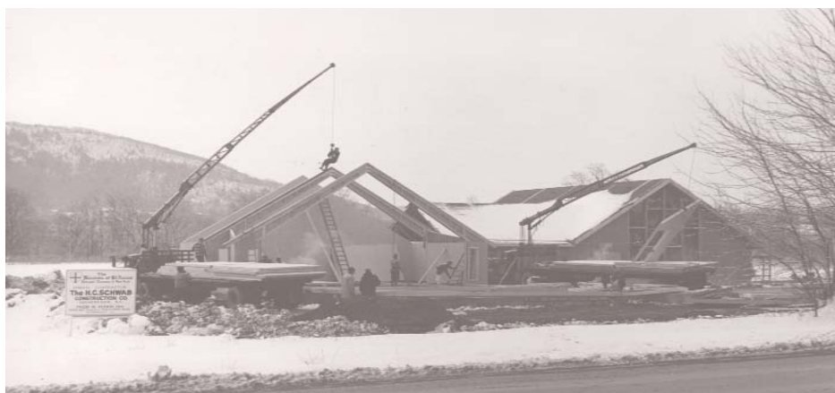
St. Anne's under construction, 1963.
