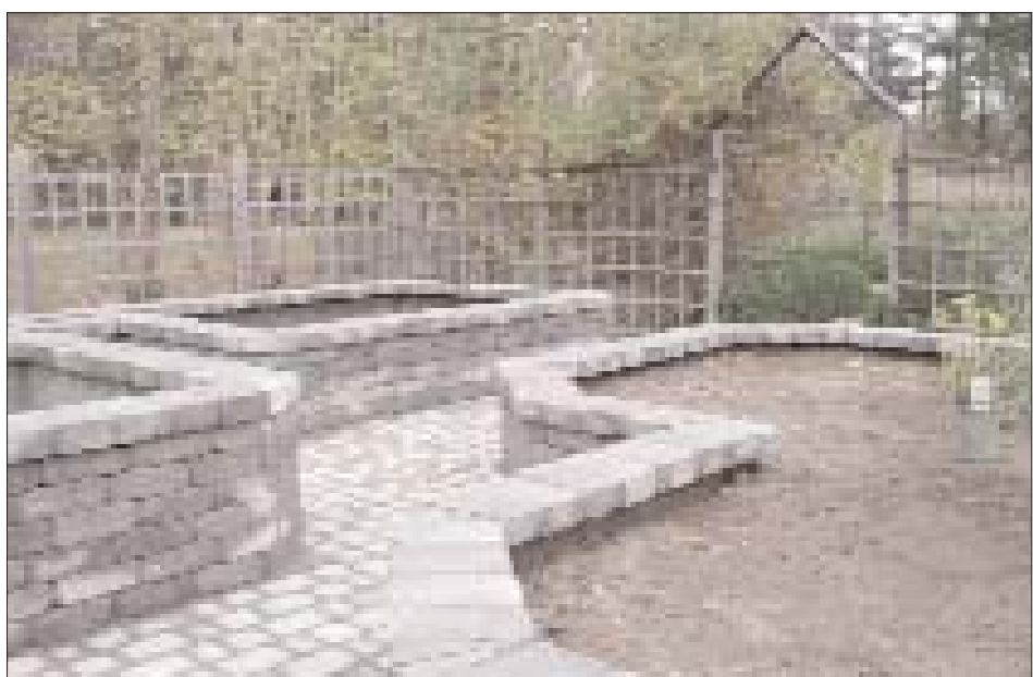
The St. Gregory's Horticultural Therapy Garden under construction.
